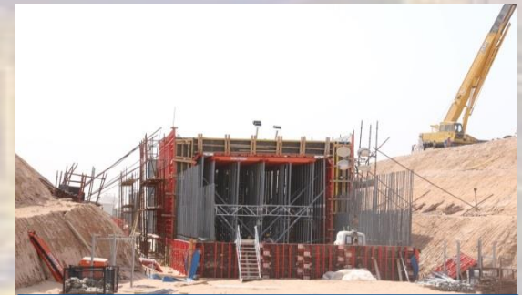
Steel Form Work
