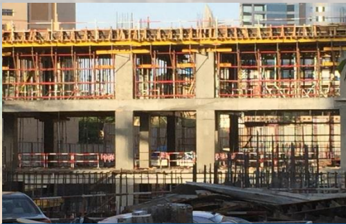
Concrete Form Work
