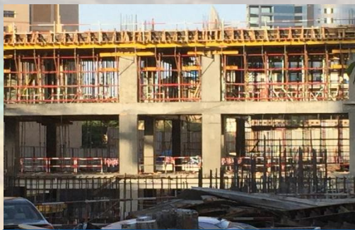
Concrete Form Work
