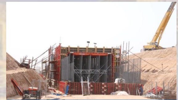
Steel Form Work
